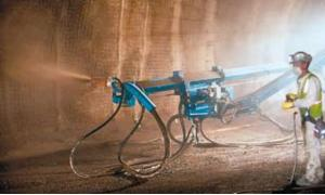
MEYCO machines are designed and built to excel in their chosen environment of tunneling, whether mounted as a spraying system on a TBM or as an autonomous mobile spraying unit.
